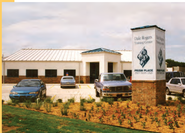
Old Meek house demolished; new building completed, housing newly created Special Needs Program for people with multiple disabilities, 1997.
