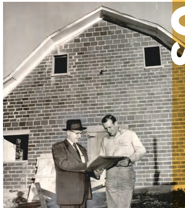
The new barn under construction in 1956, later decimated during a tornado in 1970. (Courtesy: The Oklahoman)
